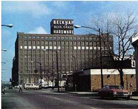
Main Offices and Showrooms 1st and Main Streets.
